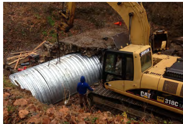
The High Falls Creek culvert sleeve.
