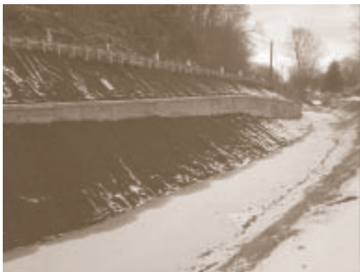
PennDOT's new wall along the Canal in Raubsville.
