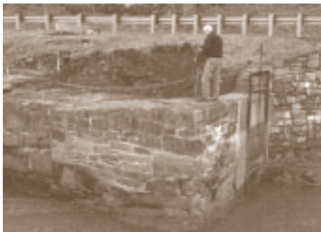
A gaping hole awaits new pipe at the Lock 20 bypass.
