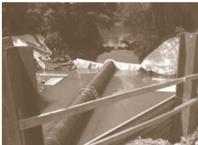
The Cuttalossa Creek construction site.
