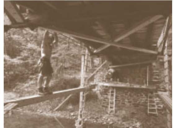
R-Shell Exteriors replaced the Hazzard's Bridge X braces.
