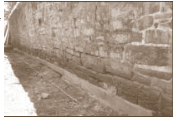
The new timber sills in Lock 18 in Uhlerstown.
