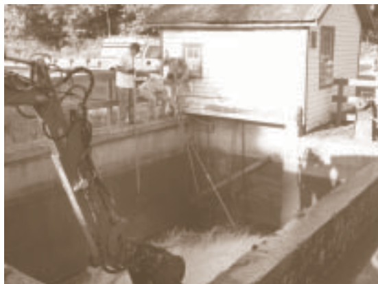
The Park staff cleans out accumulated debris from the wickets at Lock 22/23 in Raubsville on a routine basis.
