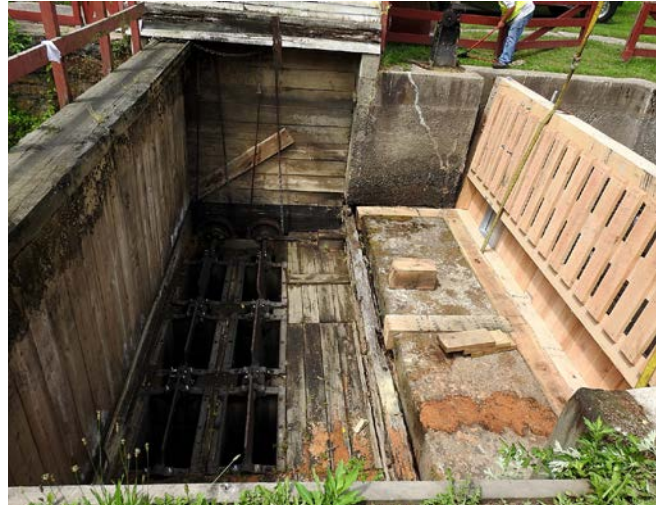
Installation of a drop gate at the Groundhog Lock. Wickets can be seen below.
