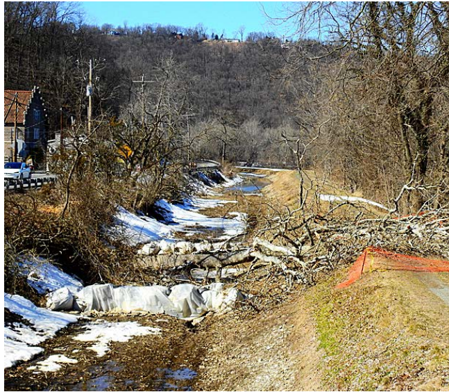
A large sycamore tree was downed at the site of the collapse north of Woody's Bridge. Its roots were undermining the Canal's prism.
