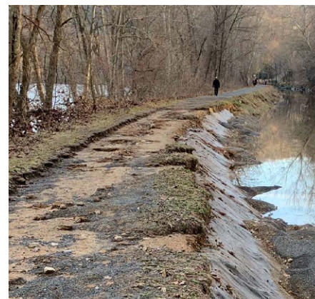
River flooding damaged the towpath banks south of Easton.
