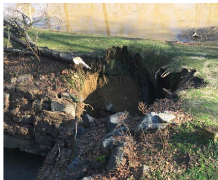
The culvert collapse in Raubsville.
