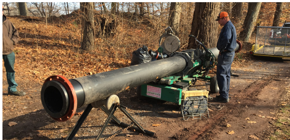
Fusing together the pieces of pipe that will carry Delaware River water into the Canal.
