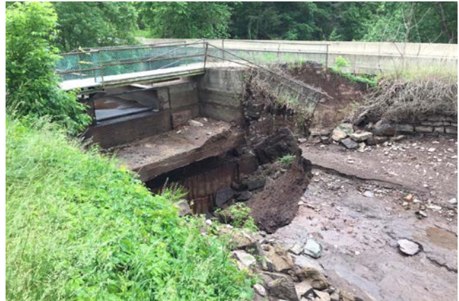
The north end of the Tincicum Aqueduct after the creek did its damage.
