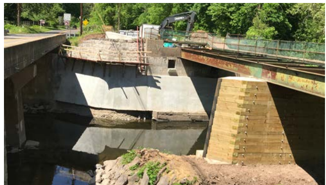
The Tincicum Aqueduct work site — June 7, 2020
