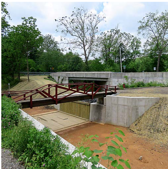
The Fry's Run Aqueduct is done. Water and growing grass will complete the picture.
