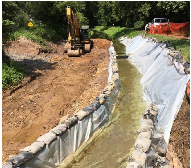
A temporary channel kept water flowing south through the Tincicum Aqueduct.
