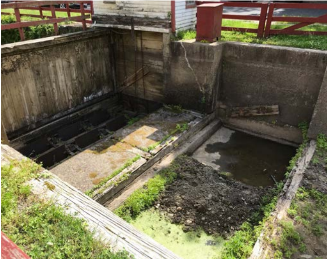
The chamber at Groundhog Lock awaits its new drop gate.
