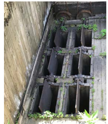
The wickets that allow water to flow into and out of a lock controlled by a drop gate aren't often in view. This replacement project offered a perfect opportunity to see them.
