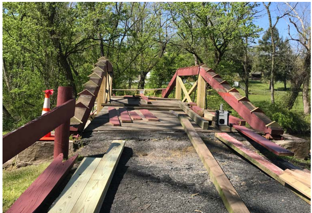
Work in progress at the Thompson-Neely Camelback Bridge.
