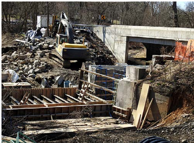
Loftus Construction in the midst of the replacement— March 8, 2020.
