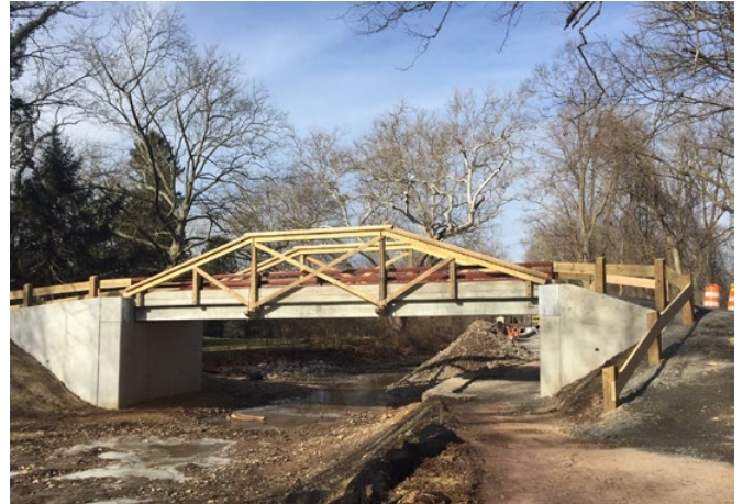
The new Phillips' Mill Bridge waiting to be red.
