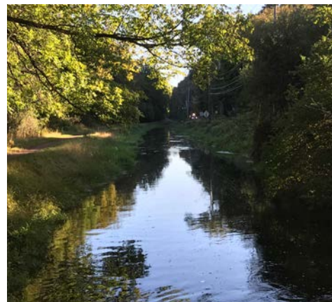
The view south from the Tinicum Aqueduct on October 5.
