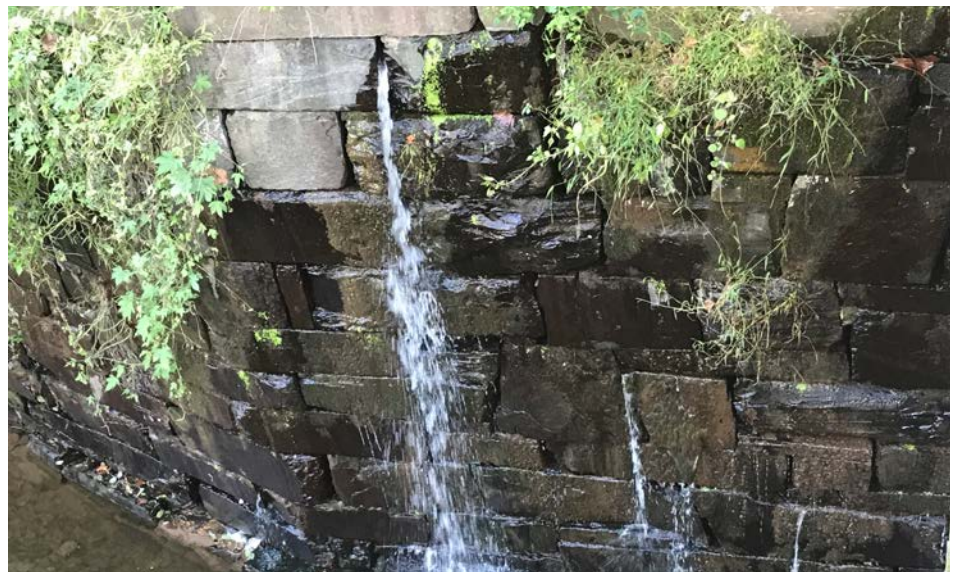
The leaks in the stone walls of the aqueduct will be plugged.
