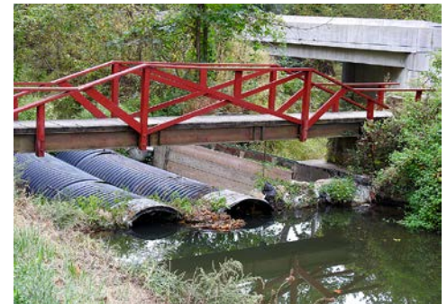
The Park has maintained canal flow by running water through temporary pipes at the failed Kleinhans Aqueduct.
