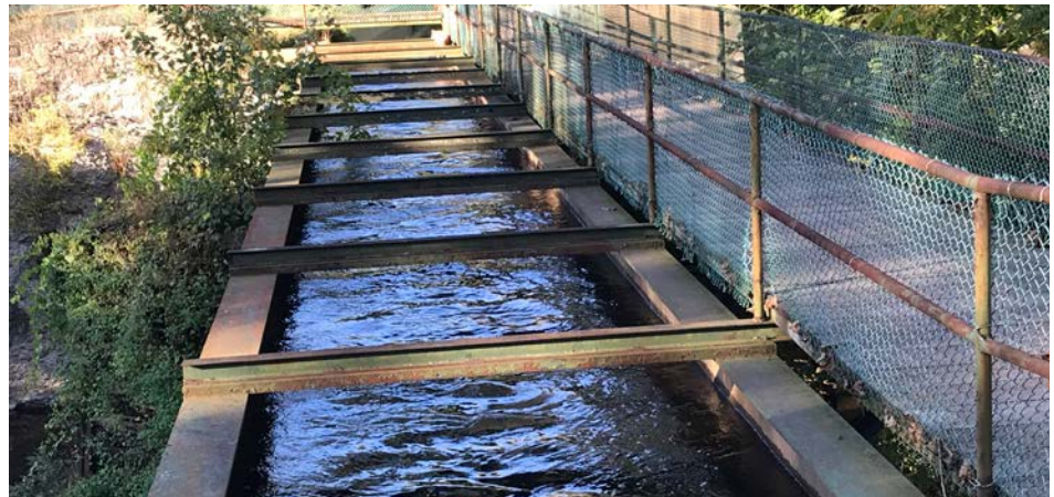
The rusting trough of the Tinicum Aqueduct will be repaired.
