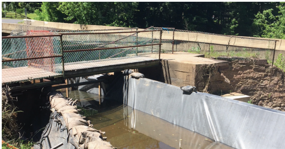
The recently widened bypass trough is conveying more water south through the Tinicum Aqueduct.
