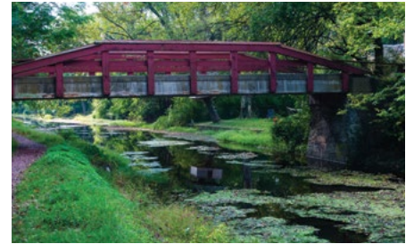
The soon-to-be replaced Phillips' Mill Bridge
