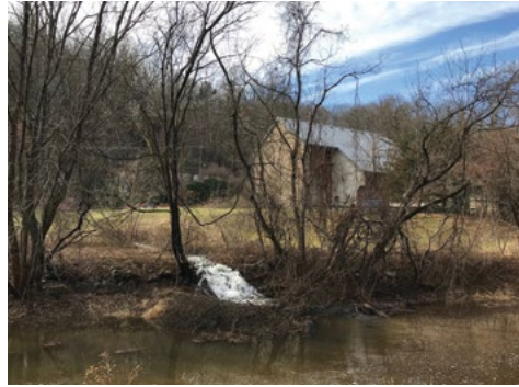
From the Point Pleasant Pumping Station to the Delaware Canal
