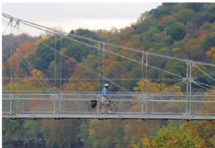
Canal looping requires crossing Delaware River bridges. WALK your bike, don't ride.
