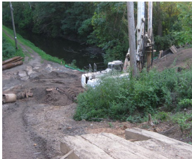
Drill rig in place on the south side of the Conrail embankment preparing to tunnel through. Photo shows the site looking down from the top of the embankment.
