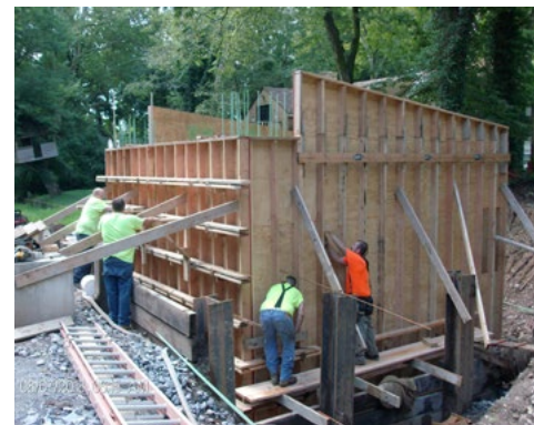
The formwork for the west abutment of the new Phillips' Mill Bridge is ready for the concrete truck to arrive.
