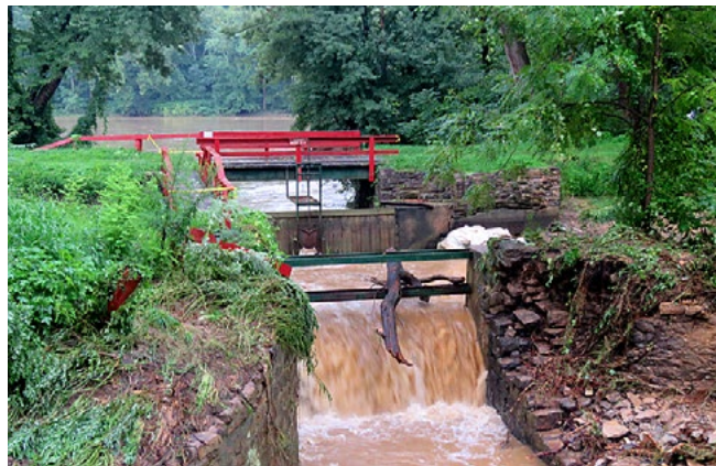
The Fry's Run Aqueduct after the August 11 flash flood. The west wall was gone and the Lehigh River poured out of the side of the remaining structure.
