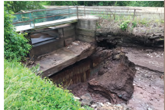
The blowout at the Tinicum Aqueduct.
