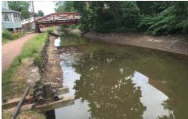
The level of the Canal in Yardley Borough on June 27, 2016.
