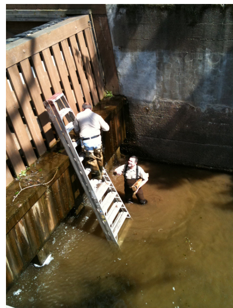
Rick van Vliet, Park Maintenance Supervisor, and Rick Dalton, Park Manager, down in Lock 11 stopping a gate leak by inserting some oakum..
