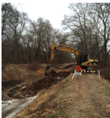
Bi-State Construction removed the coffer dam north of the culvert project allowing Lehigh River water to flow south.
