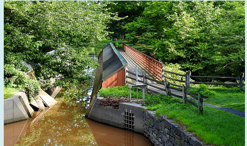
Tohickon Aqueduct in Point Pleasant Mile 32.750
