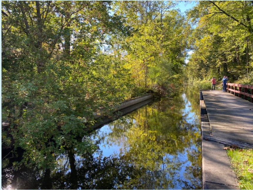
Gallow's Run Aqueduct in Kintnersville Mile 47.162
