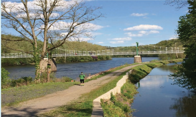
Pedestrian Bridge linking PA to NJ in Lumberville Mile 30.914
